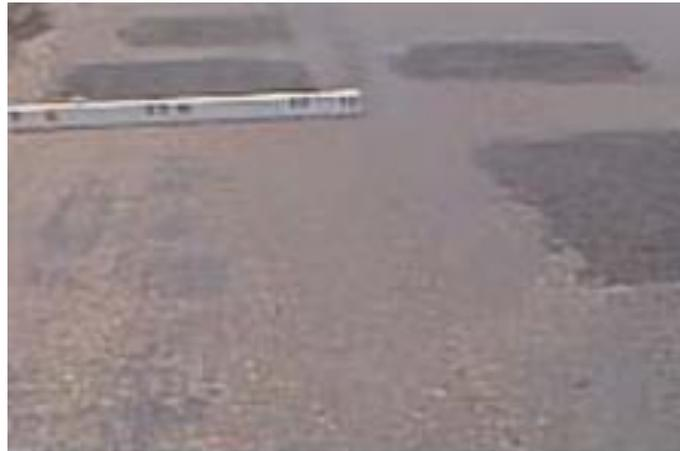
Gambar 12. *Patching and Utility Cut Patching* (Sumber: Internet, 2022)
